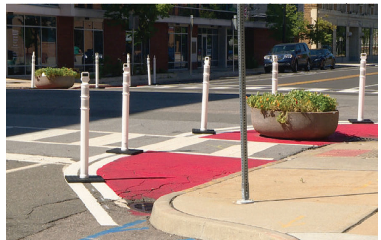
Example of curb extension with tubular delineation.
